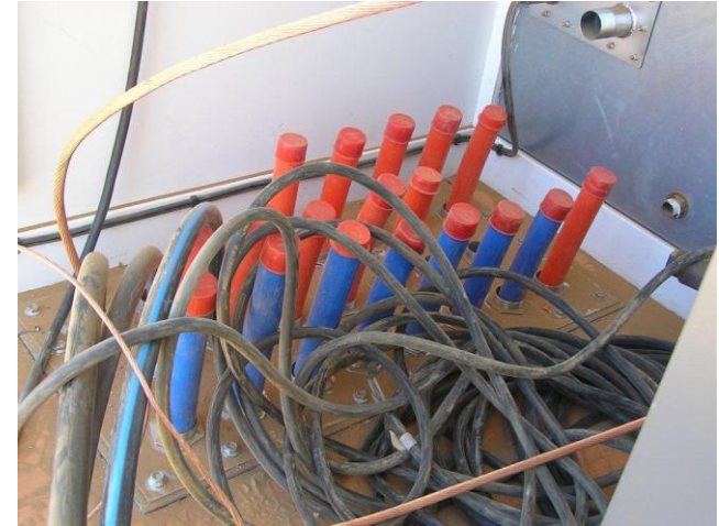
Colour-coded subducts during installation
