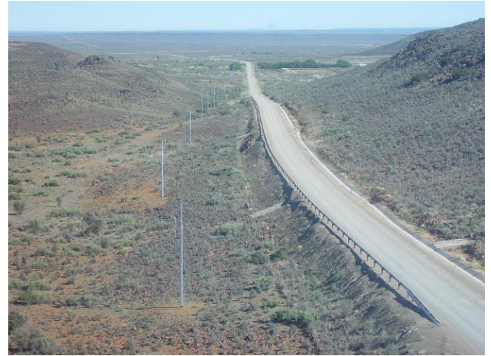
New 33 kV Powerline with MASS fibre optic cable approaching Core Site
