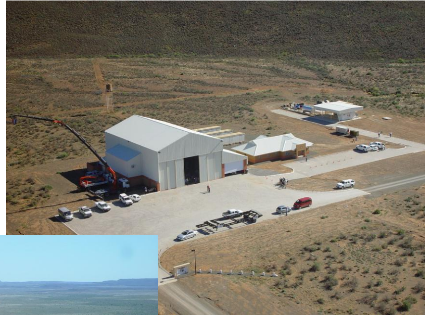
Core Site Complex
