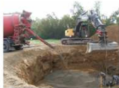
Soil exchange at location 2
