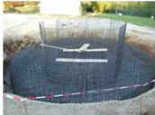
Basement armor of the concrete towers
