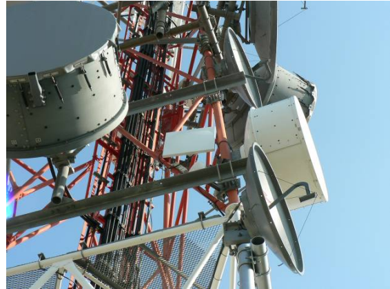
Fig. 3. Square-shaped WiMAX antenna at the Gardunha relay tower (relay stations are mounted back-to-back).
