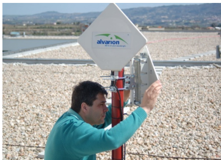
Fig. 8. Fine tuning of the WiMAX antenna tilt.
